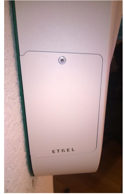
Figure 55: Secure maintenance doors enclosure using hex key
