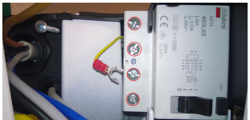
Figure 39: Check that the marked screws are unscrewed so that wires can be inserted
