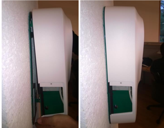
Figure 52: Attach the charging station to the top hooks and push it to the wall
