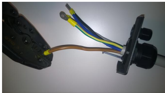
Figure 27: Squeezing the ferrules of the wiring
