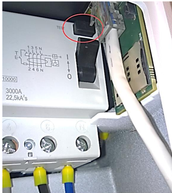
Figure 43: RCD test button
