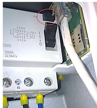
Figure 39: RCD test button
