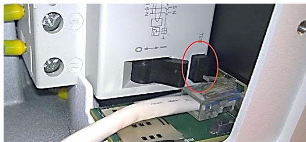
Figure 34: RCD test button
