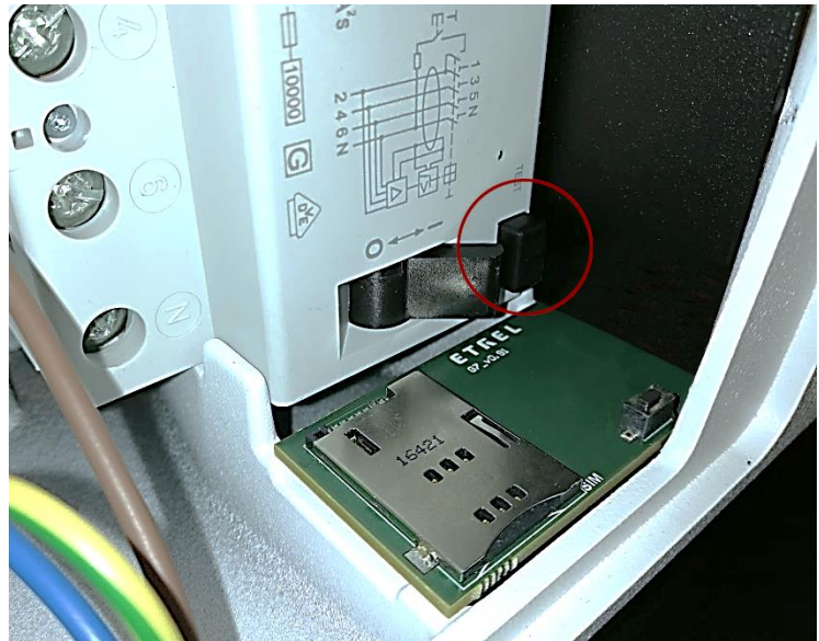
Figure 5: Bouton de test RCD
