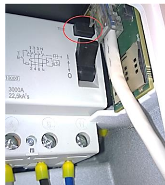
Figure 9: RCD test button
